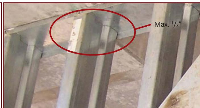
Load bearing walls are designed to fully seat within the top and bottom tracks. Design standards recommend a maximum gap of  $\frac{1}{8}$ " in order to obtain an effective bearing condition.
