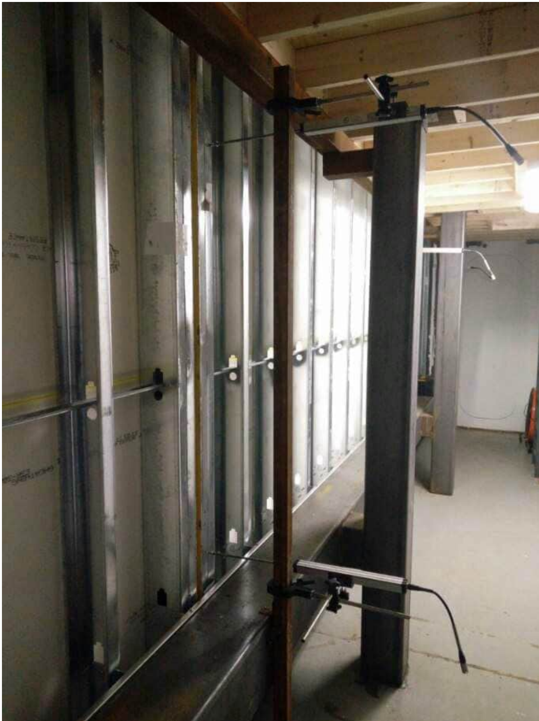
Photo B20: Linear displacement transducer location for structural testing
