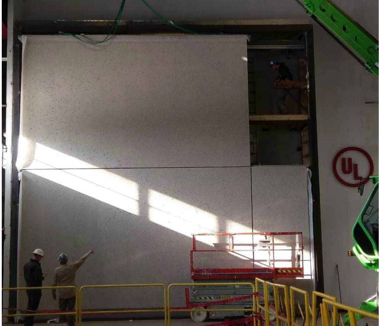
Photo A20: Second row of panel installed
