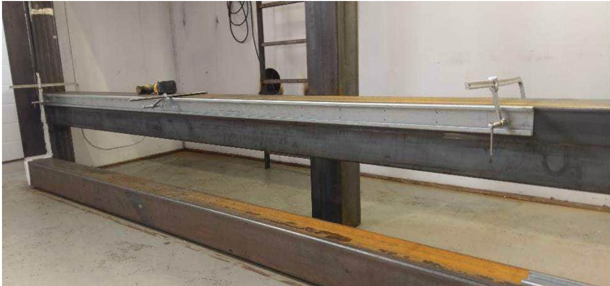
Photo A5: "DriftTrack®" installation along horizontal members
