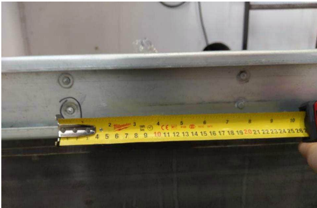
Photo A6: "DriftTrack®" Installation with rivet nails at nominal 178mm (7") C/C
