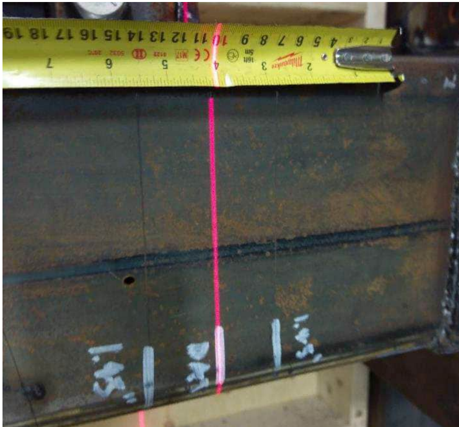
Photo B15: Interstory horizontal (in/out) movement test reference datum
