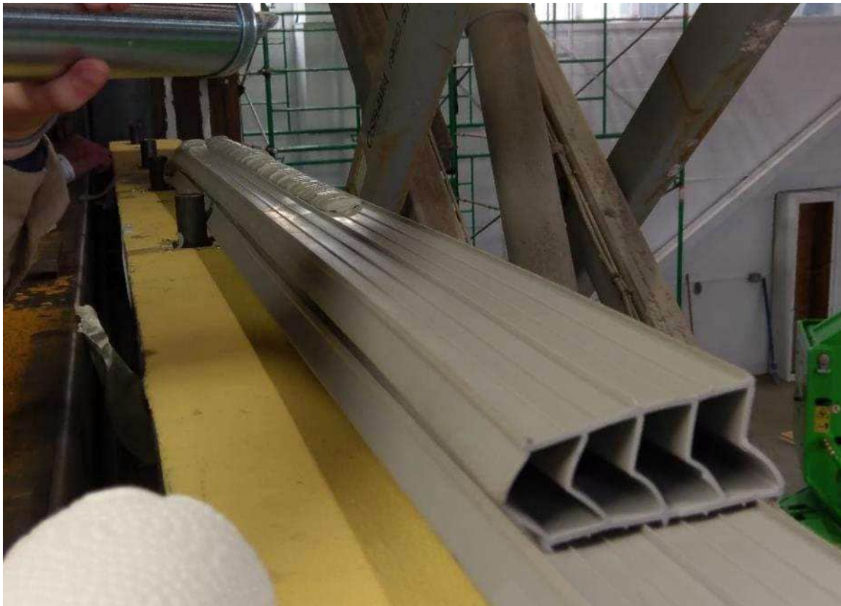
Photo A16: Sealant application at the horizontal panel to panel gasket
