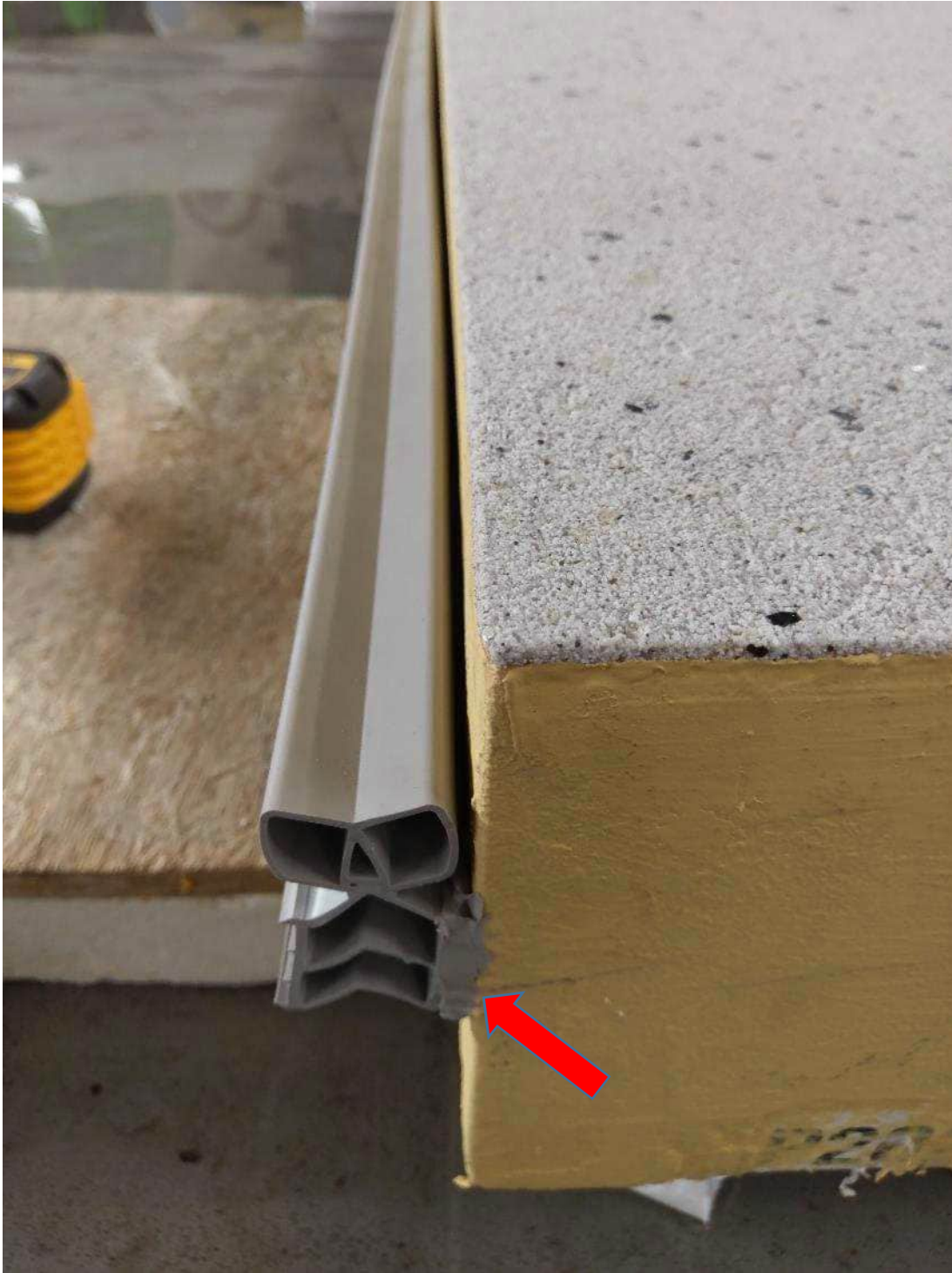
Photo A10: Pre-installed panel to panel gasket sealed with Dow 795 sealant detail
