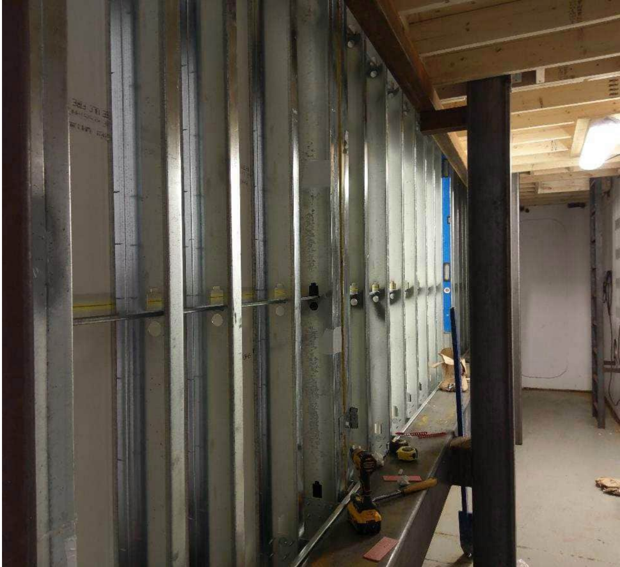
Photo A14: First row of panels as shown from interior side
