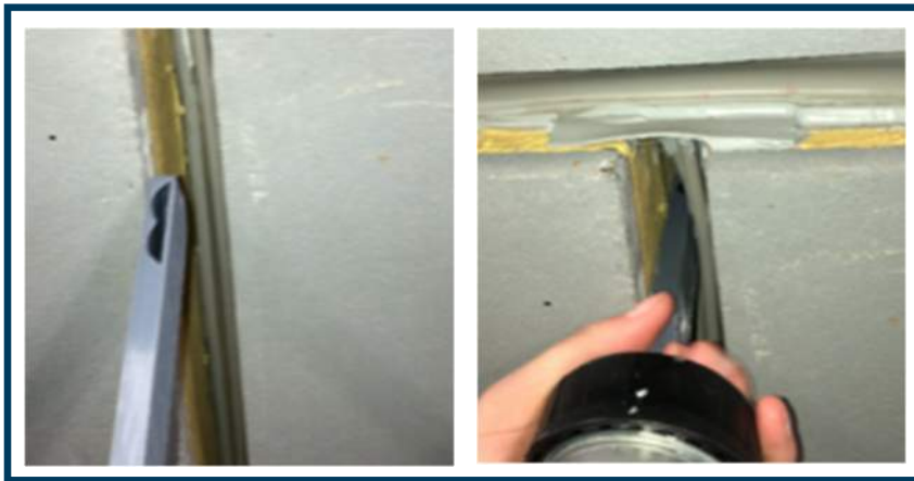
Whistle Tips for installing sealant IN-PLACE
